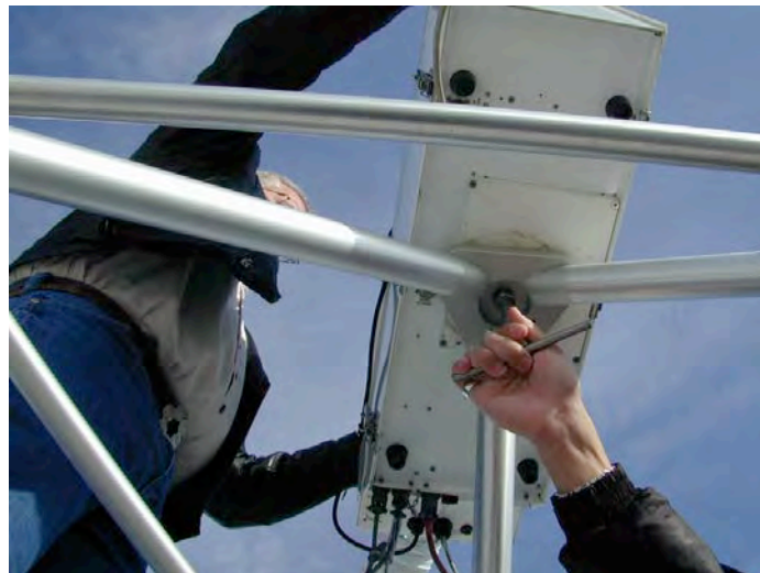
Figure 3-4. Securing the profiling radiometer with the T-Bolt
