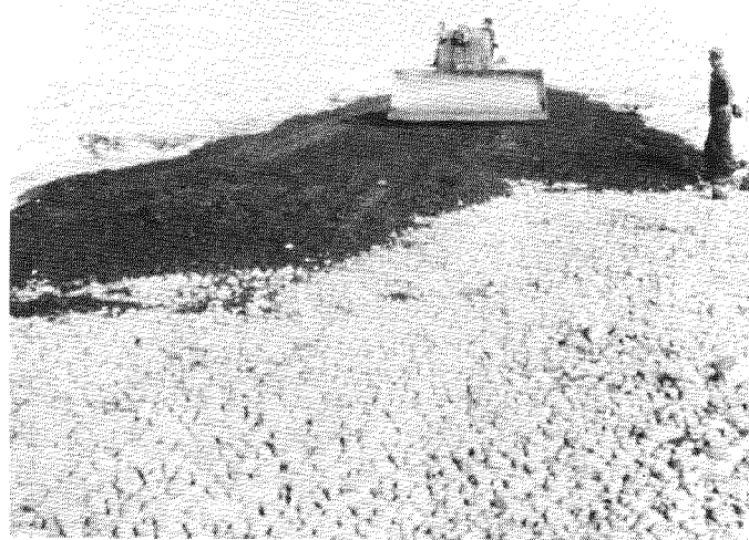
Fig. 3. Bulldozers spreading and compacting fill
