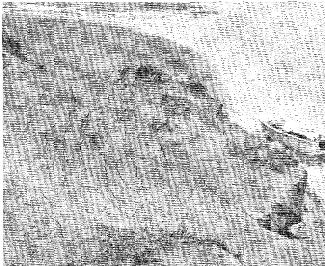
Fig. 15. Tension cracks in top of sand dune over the thermo-erosional niche in Fig. 13
