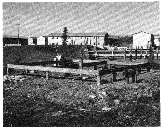
Fig. 4. Pile foundations for house.
