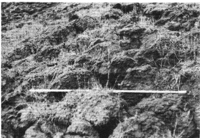
Fig. 2. Widened cracks and fully developed clay hummocks
