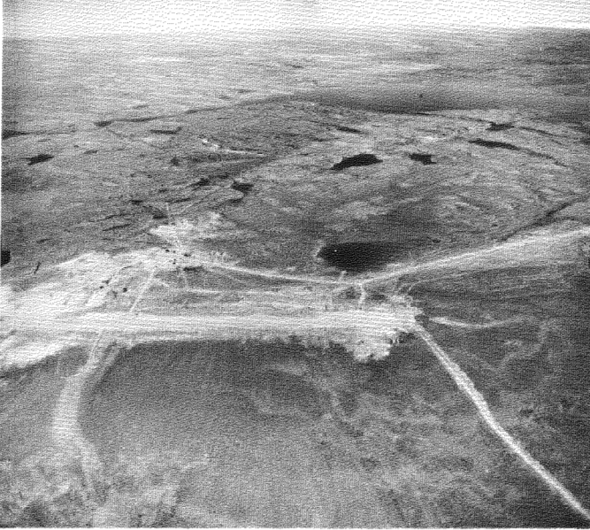
Fig. 2. Station in Melville Peninsula. Note development of airstrip on slope. Soil flow is indicated by striping
