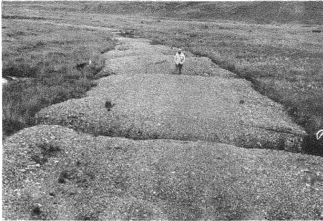
Fig. 5. Roadway destroyed by thawing of ice-wedge tops at Umiat, Alaska. Gravel fill was not thick enough to replace insulating effect of the organic mat which it destroyed (photo by Gordon W. Greene)
