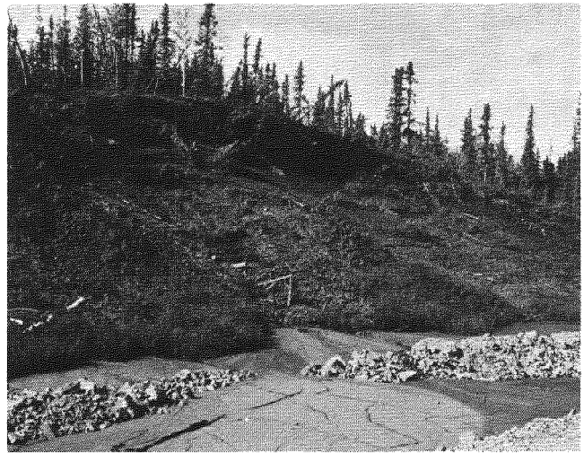
FIGURE 8 Desiccation of ditch sediments and continued slope recession, 31.6 km, 17 August 1971.
