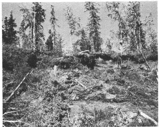
FIGURE 17 Untidy appearance and continued thawing of backslope, 32.6 km, 17 August 1971.
