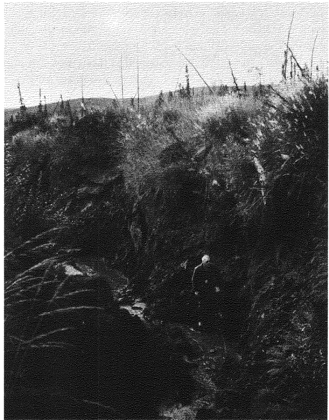
FIGURE 1 Gully erosion resulting from fireline construction in ice-rich permafrost soils.
