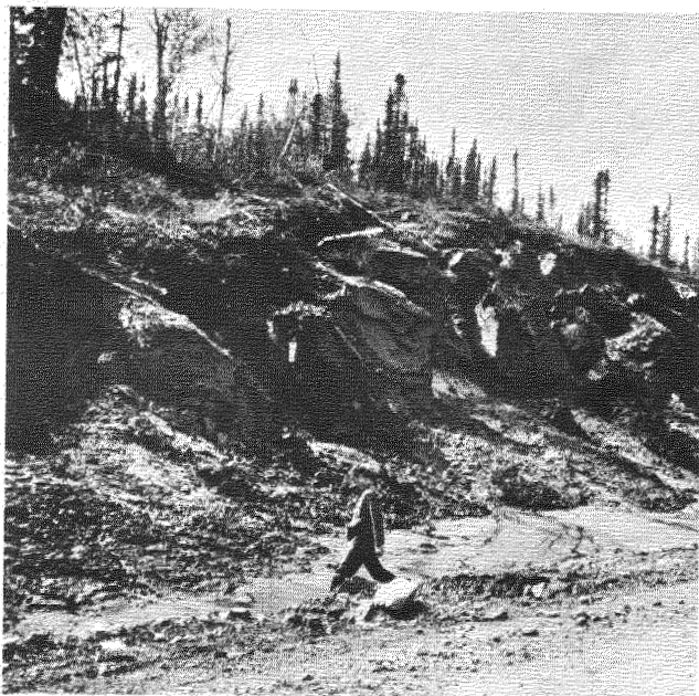
FIGURE 4 Thawing backslope, 31.6 km, 26 June 1970.
