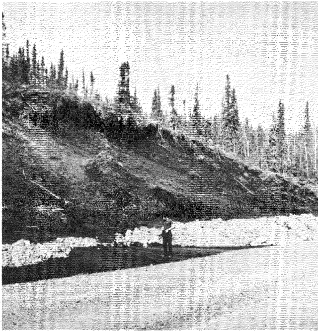
FIGURE 7 Receding backslopes and stabilized ditch sediments, 31.6 km, 28 May 1971.
