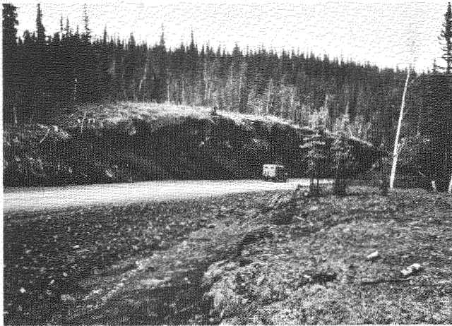
FIGURE 11 Overhanging mat and clearing atop backslope, 32.6 km, 26 June 1970.
