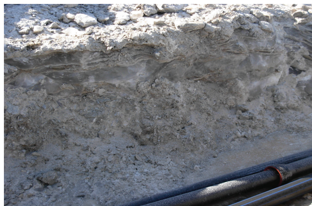
Figure 1. Ground ice of the rock glacier with water conduit for artificial snow production (lower right).
