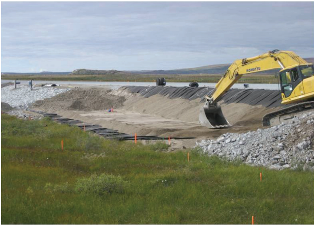
Figure 1. Installation of the heat drain in the shoulder of the Tasiujaq airstrip embankment.
