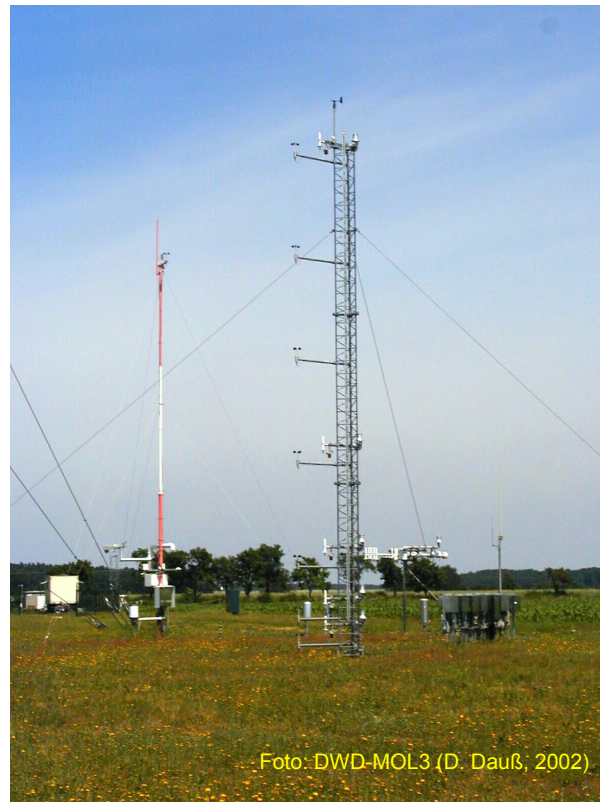
Figure 5 The 10 m mast for standard meteorological measurements from SSW
