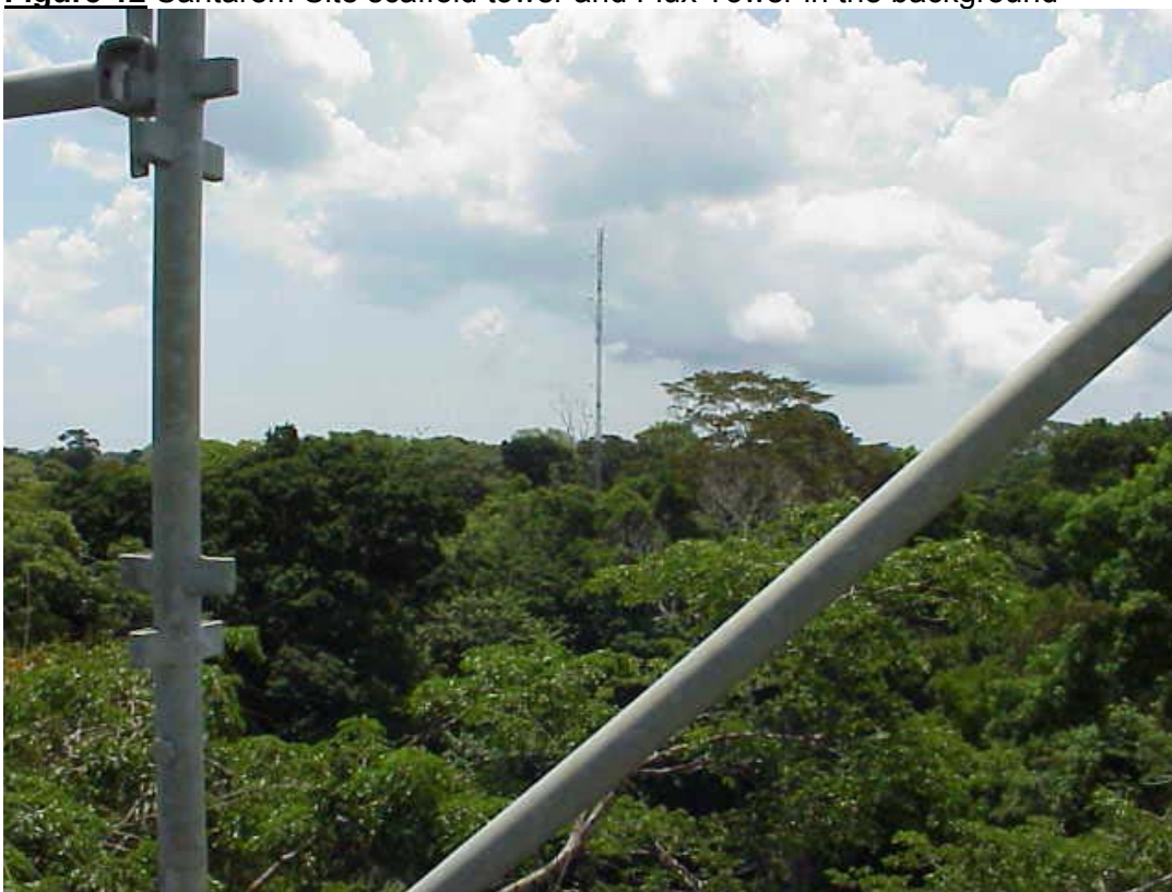
Figure 12 Santarem Site scaffold tower and Flux Tower in the background
