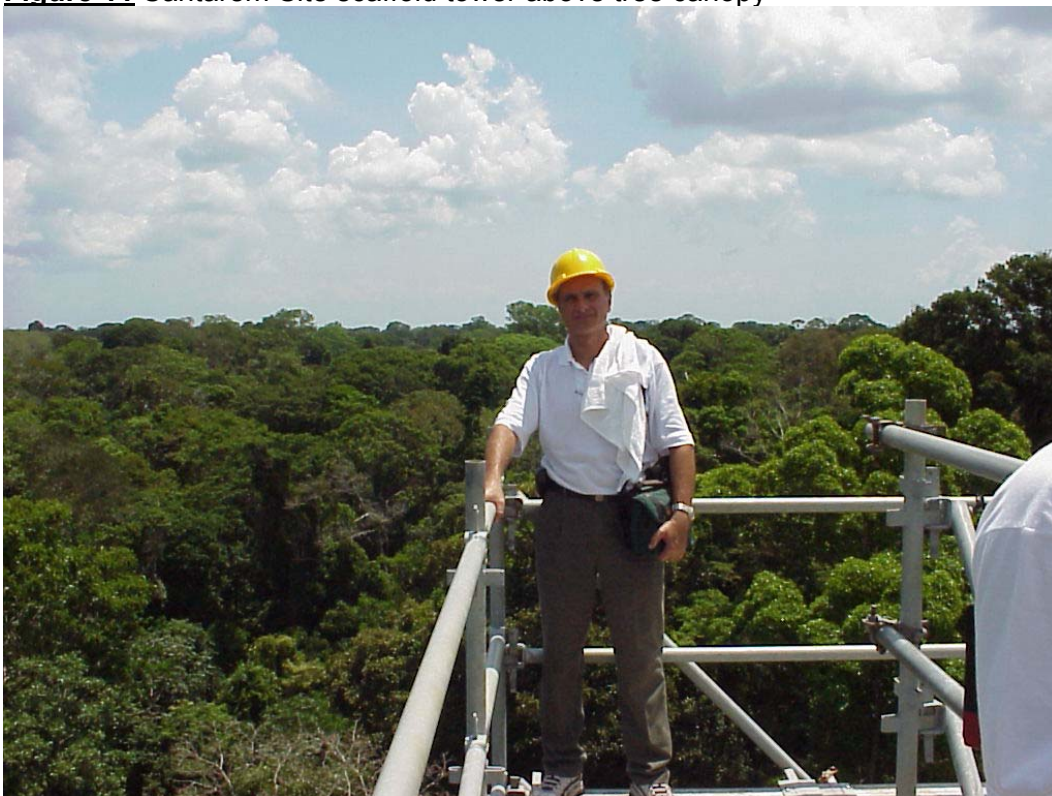
Figure 11 Santarem Site scaffold tower above tree canopy
