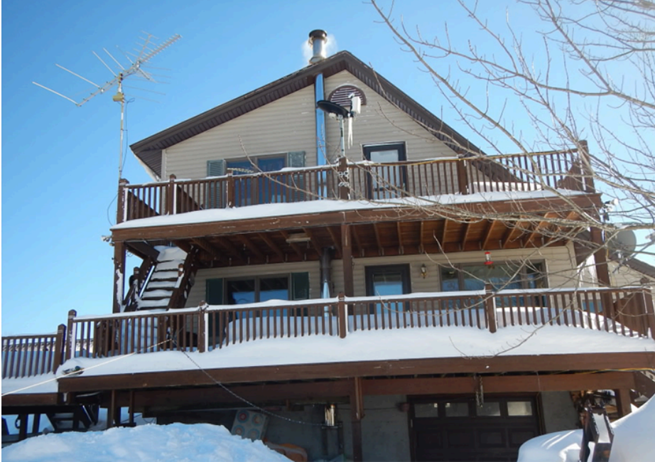
Looking East at North Redfield site
