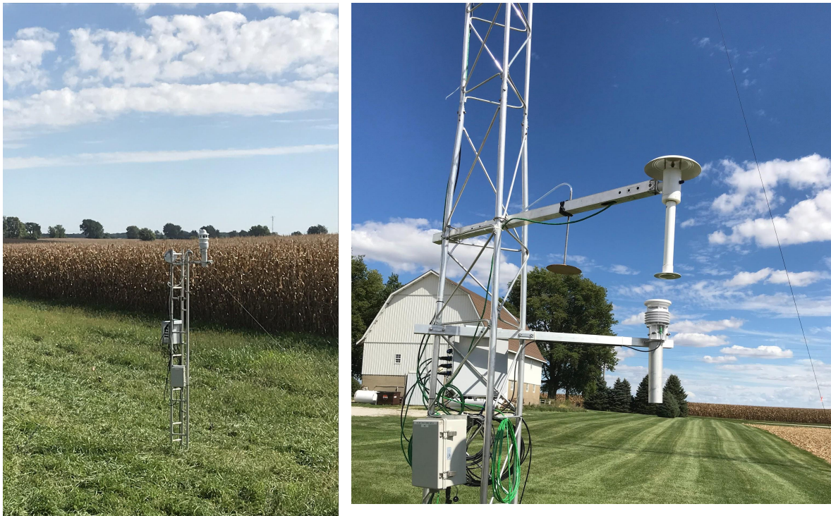
Figure 2: (left) Vaisala PTB. (right) ISFS Temp/RH sensor (top) and Lufft WS300 (bottom).
