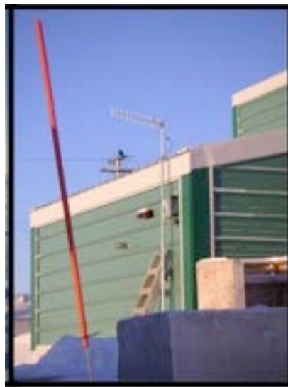
Figure 21: DFO garage where line of sight receiving antenna was located to data transfer.
