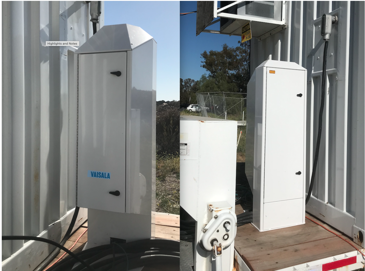
Photo 1. SB Fire Dept site where the Vaisala CL61 was deployed.
