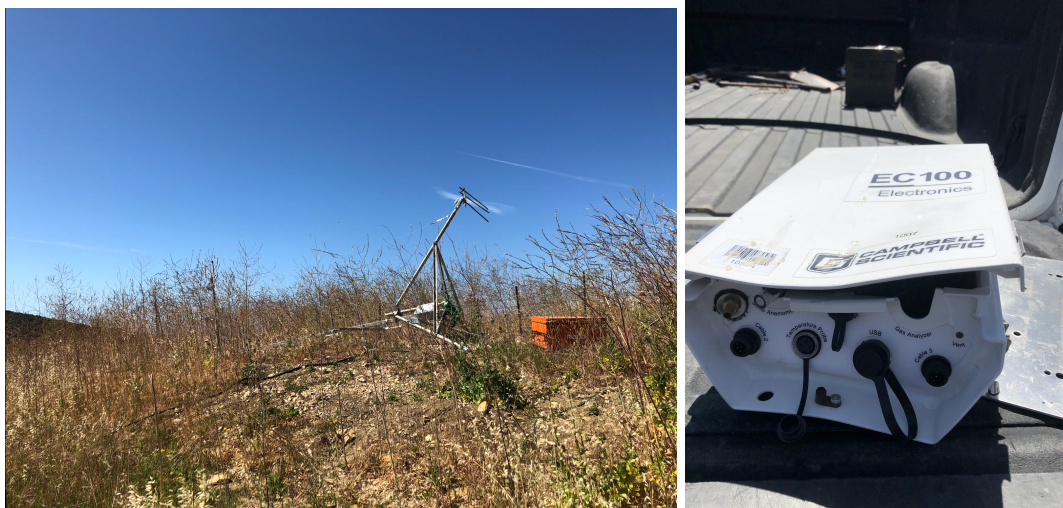
Photo 3. Site 5 showing the fallen tower (left) after high winds blew it down. The stakes on the “northwest” leg were pulled from the fairly loose, sandy soil. Upon visual inspection the only damage was to the EC100 (right), which was dented after landing on a rock. The re-elevated mast was resecured with a 70 pound bag of sand on each tripod leg.
