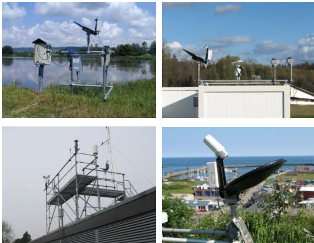
Figure 8: Examples of MRR installations
